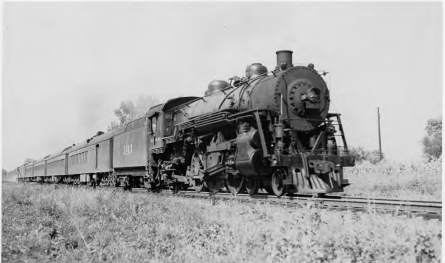
Pacific #1143 and train in Central Illinois. The window arrangement and unique air conditioning roof hatch indicate that the first car is car #890, #893, or #894, a 76'5" Baggage-Smoker. Paul Stringham photo
