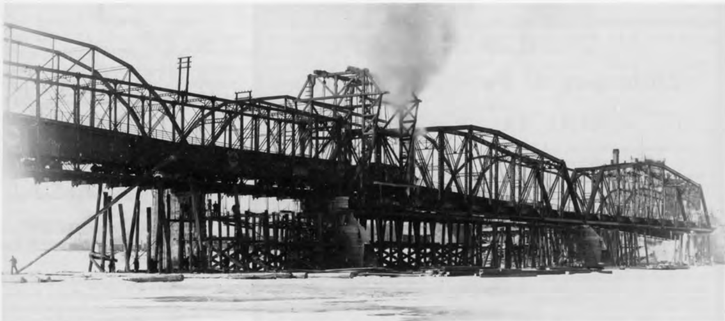
Rebuilding of the Mississippi River bridge at Dubuque. View west from the north side of bridge. Carriage "High Bridge" can be seen behind the Railroad bridge. ICRR photo.
