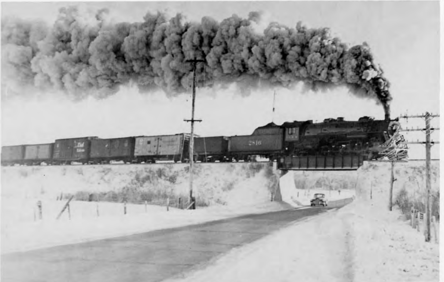
#2816 eastbound crossing US route 20 approaching Freeport Illinois. W.L. Heitter photo.
