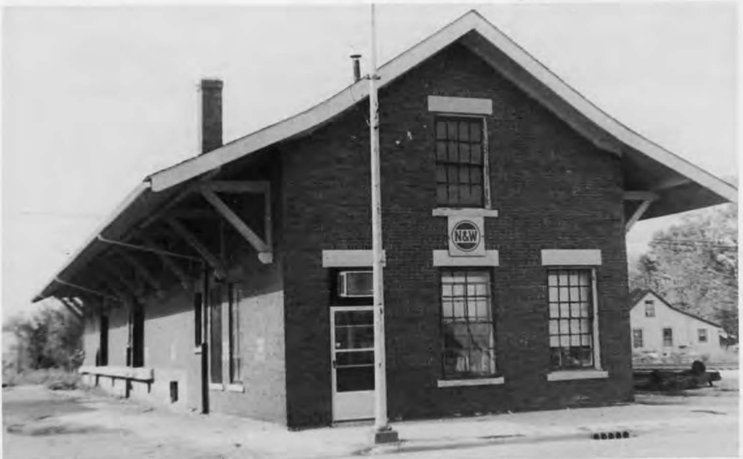
The Paxton, IL Norfolk Southern freighthouse - soon to be ICBS headquarters building.
