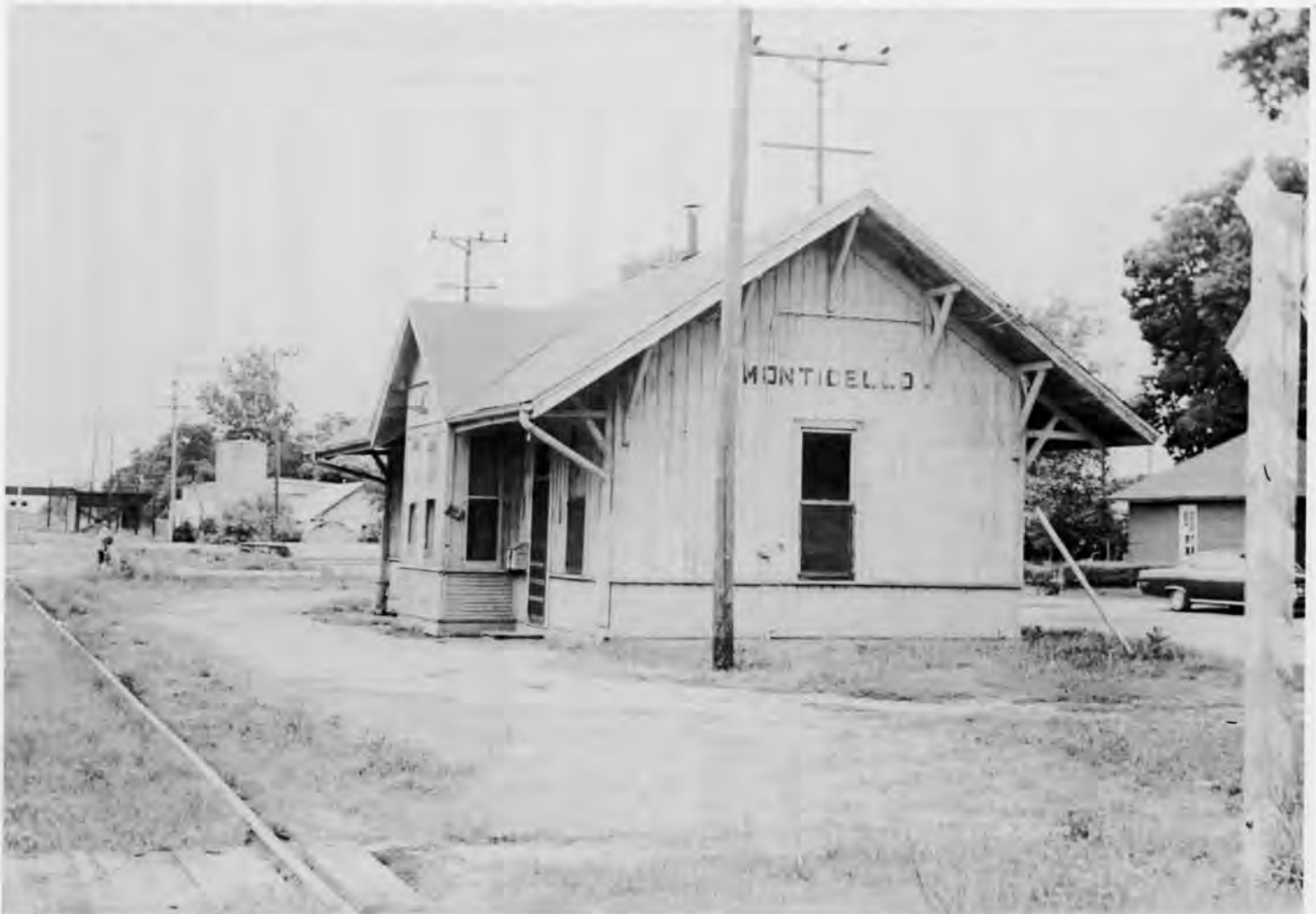
The Monticello depot (on the Champaign - Decatur line) is a type "A" with a single waiting room, but it has both a window and a door at the front of the waiting room similar to type "D" depots, but only 1 window in the waiting room end of the building. This depot may not have been rebuilt, note the oversize roof and large eaves. W.C. Thurman photo.
