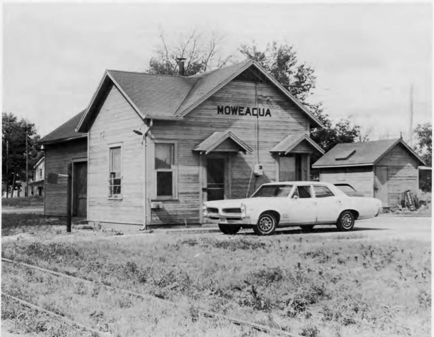
The Moweagua depot (south of Decatur on the I.C. charter line) shows a typical type "B" depot with two end doors at the office end of the building. The shed behind the depot is similar to a type "C" freight room. Also note the "modern" train order board in use after the original semaphore type train order signal was removed. (It's the flag on the short post in front of the window. W.C. Thurman photo.
