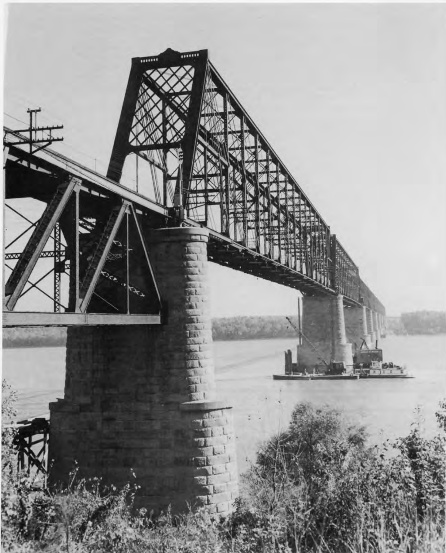
A view of the original Cairo bridge looking east across the Ohio River from the Illinois side of the bridge. Note the curve to the south at the far end of the main bridge spans as the track swings to the right into Kentucky. Also notice the signal head turned to the side at the first span. The Cairo bridge was featured in color on the cover of our 1990 calendar.
