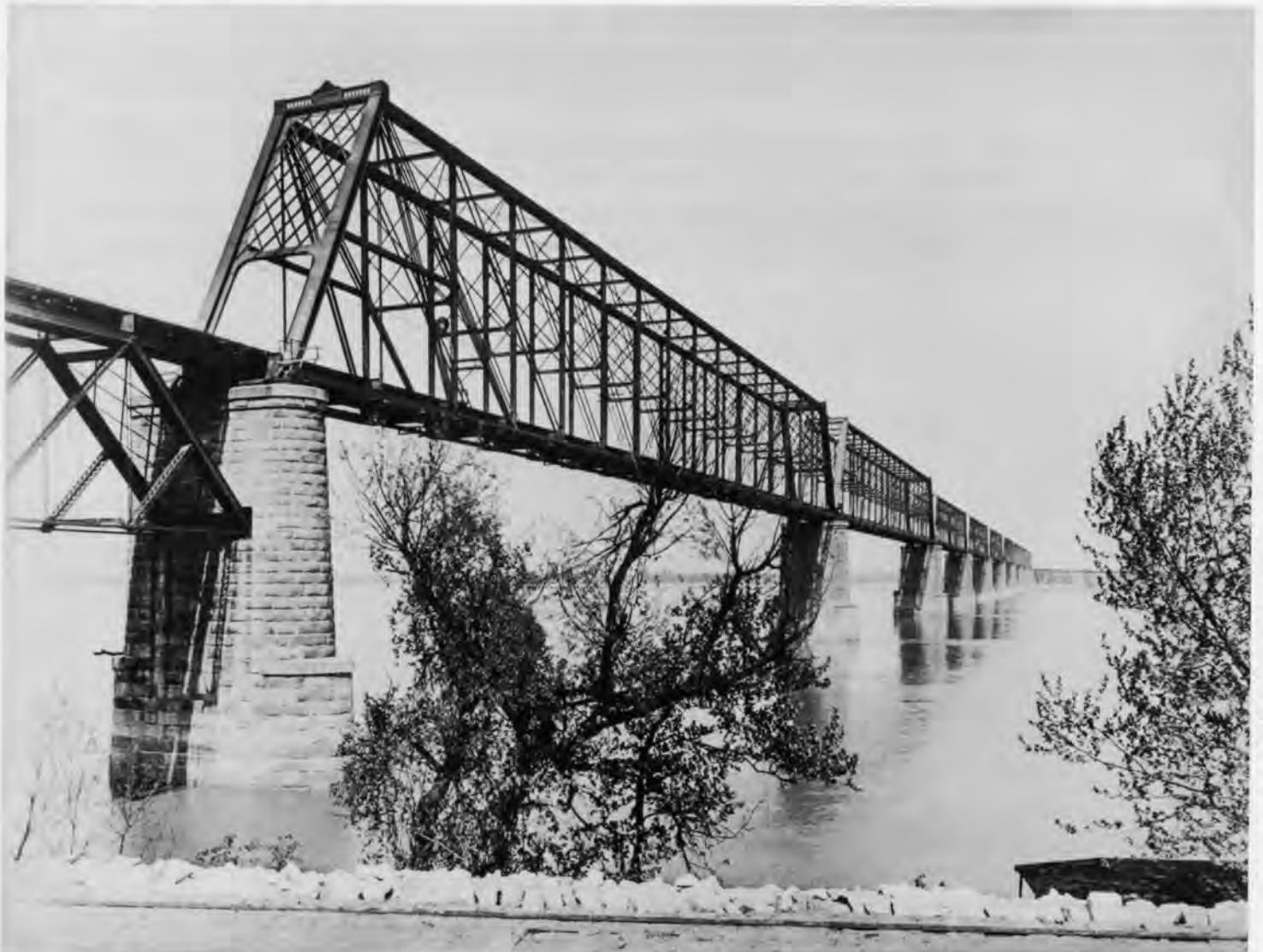
An older view of the bridge shows the much lighter construction of the first approach span. Compare this photo to the one at the beginning of the article. ICRR photo.
