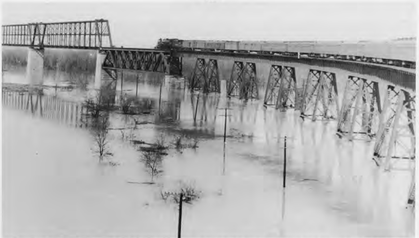
This view of a passenger train northbound on the Cairo bridge shows the steel trestles along the curve on the Kentucky side of the Ohio river. This photo also shows why the approaches were built so high leading to the bridge. During flood season the Ohio and Mississippi rivers tend to overflow their banks. ICRR photo.
