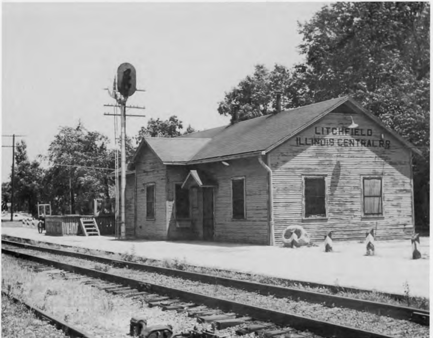
Litchfield Ill. depot is a type "D" design with a single large waiting room (near end). Note the high loading platform at the far end of the building to facilitate easy loading and unloading of freight at train level. (also trucks & wagons from the depot) Photo by W.C. Thurman 6-68.
