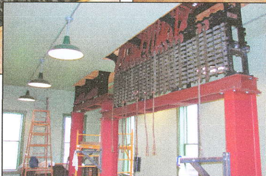
Above; Progress is being made with the installation of the levers from the IC Gibson City Tower.
