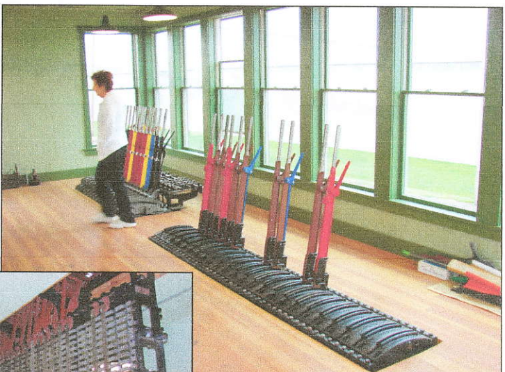
Above; Progress is being made with the installation of the levers from the IC Gibson City Tower.
