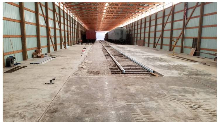
Right: The concrete floor has been poured for the new shop complex inside the car storage building. The track has been extended into the shop area for convenience of working on a piece of equipment.
