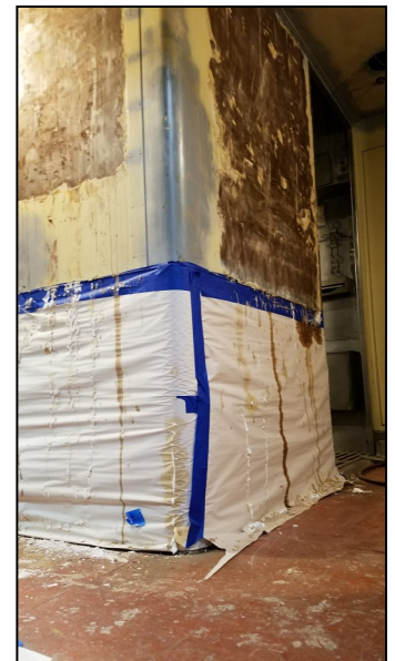
Interior wall with chemical stripping applied. Dale Jenkins Photo
