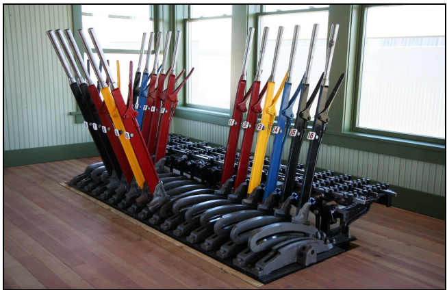
The installation of the first set of levers. Dave Marshall photos
